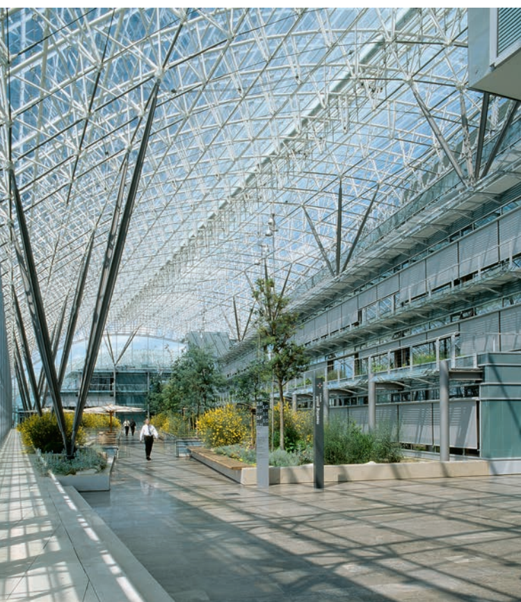
Roof glazing with spherical plain bearings
